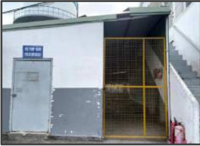
FIRE PUMP STATION
